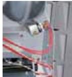
**Safe** Temperature limit control, reliable gas valve and induced draft motor plus a patented draft safety switch that shuts off the furnace if a vent blockage is detected.
